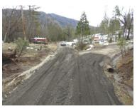
created to assist the flow of water away from Cascadel Road as well as some culvert clearing.
